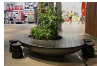
Custom Seating Unit A custom timber deck and tinted sealant was specified
